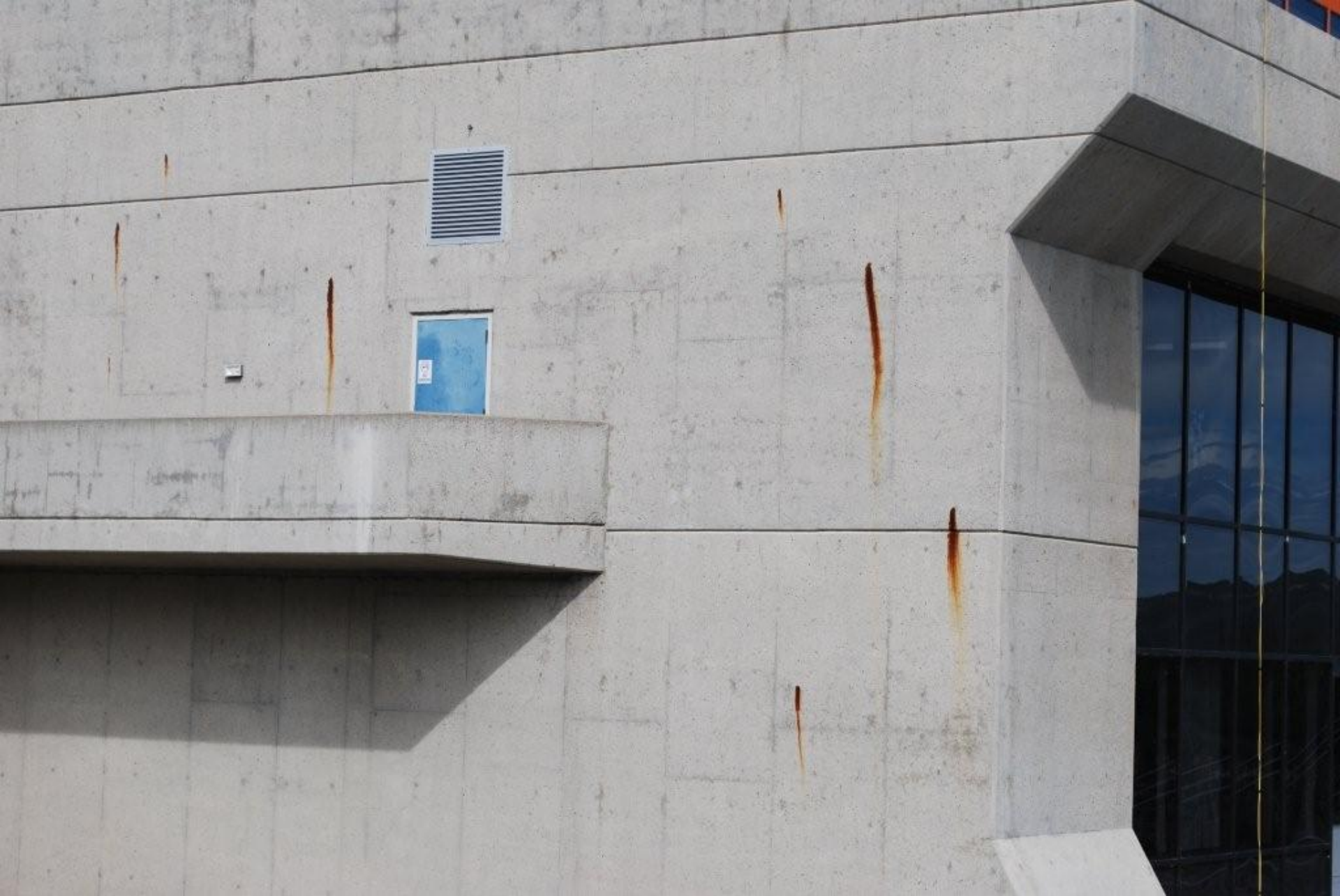
Iron sulphide stains, Peace Canyon Dam, Peace River, Northern BC, 2011
