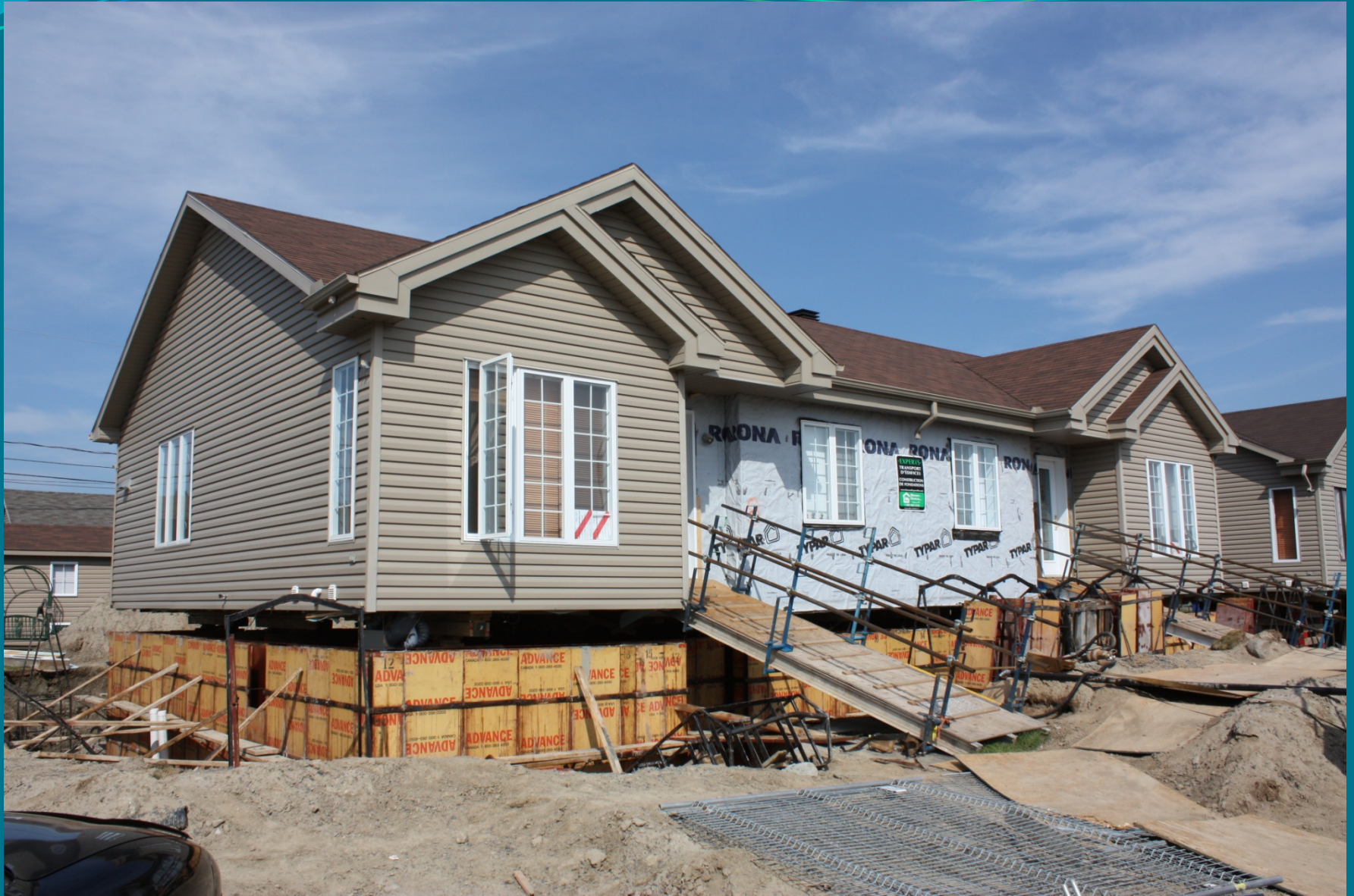
House jacked up to replace concrete foundation
