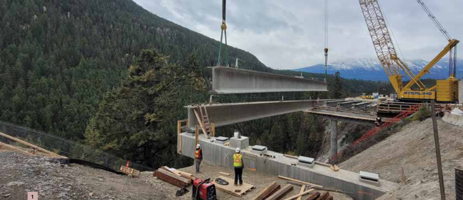
1. 42 metre long NU girders being installed at the Kicking Horse Canyon Sheep Bridge. Ten new girders were installed in three days. / Il a fallu approximativement trois jours pour poser dix poutres NU de béton préfabriqué.
